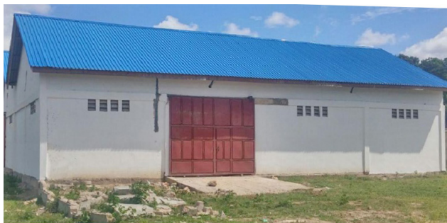
Figure 7. WLABs in a covered storage shed in Tanzania (Courtesy of Phenix Recycling).
