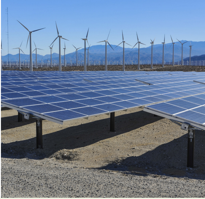
Lead-based batteries are used for large scale energy storage for renewable energy sources
